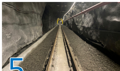
Backfill side of track for walk ways
