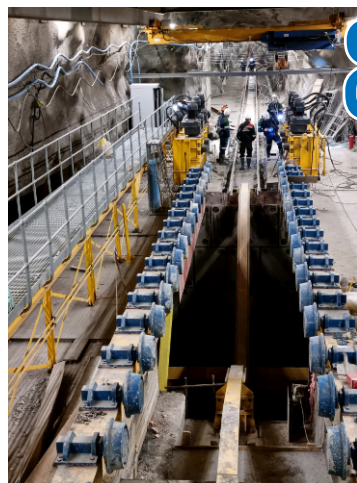
Backfill side of track for walk ways
