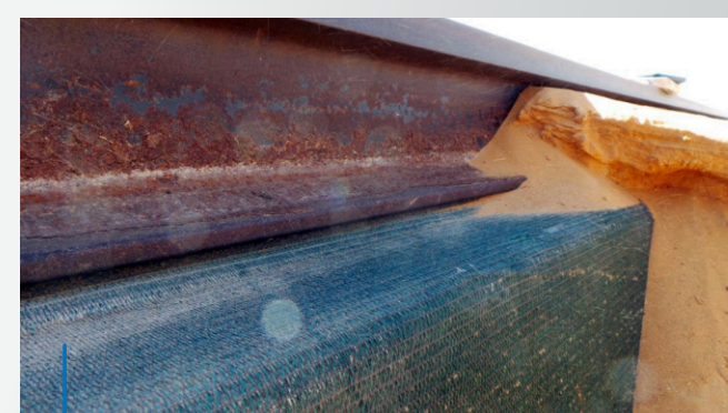
Resilient pad between rail and beam – no ingress of sand
